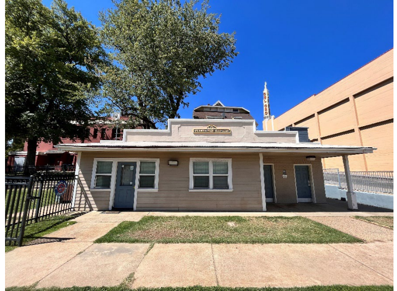
Front of Building
