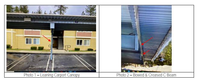
Based on provided information, our office believes significant snow loading damaged the carport structures inducing deformed and buckled structural light-gage framing members. Once light-gage members experience deformation (i.e., flange and web crippling) their structural integrity is greatly compromised, and they should be replaced. In our opinion, snow loading damaged the carport structures located at 265 Sutton Way, which now require replacement.
