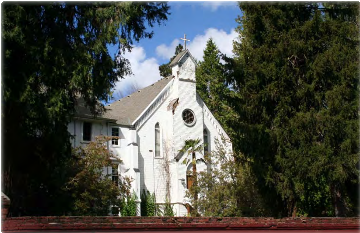
Mount St. Mary's Convent Gothic Revival Church. Note the rose window below the gabled spire and above the main entrance door.
