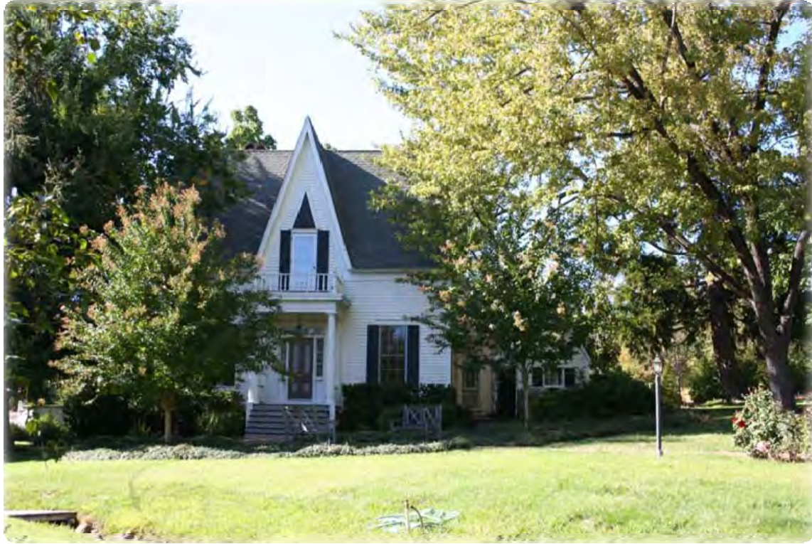
Gothic Revival Residence lacking icicles in the central gable, but exhibiting classic Carpenter Gothic design elements, such as the steep front facing cross-gable roof.
