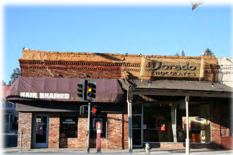
Pair of circa 1850s commercial storefronts with altered door entrances.
