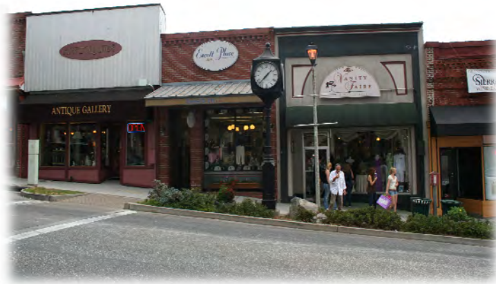
Row of brick storefronts with flat parapets of different heights facing W. Main Street.
