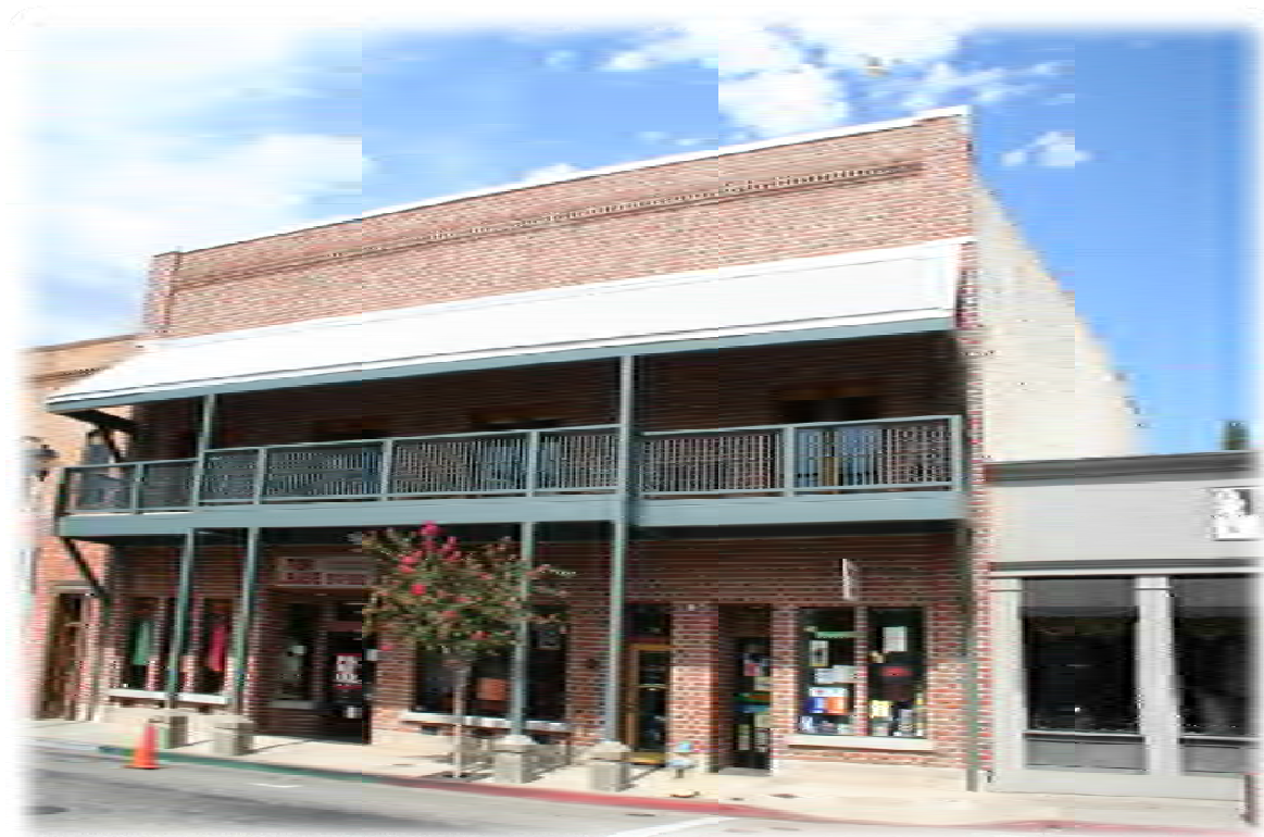
Rehabilitated commercial storefront facing E. Main Street.
