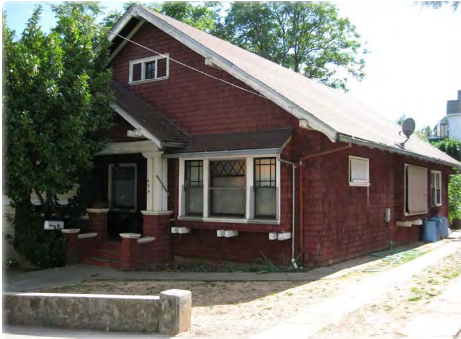
Another front gable Craftsman with shingle exterior cladding. The triple window with divided sashes typifies this house type.
