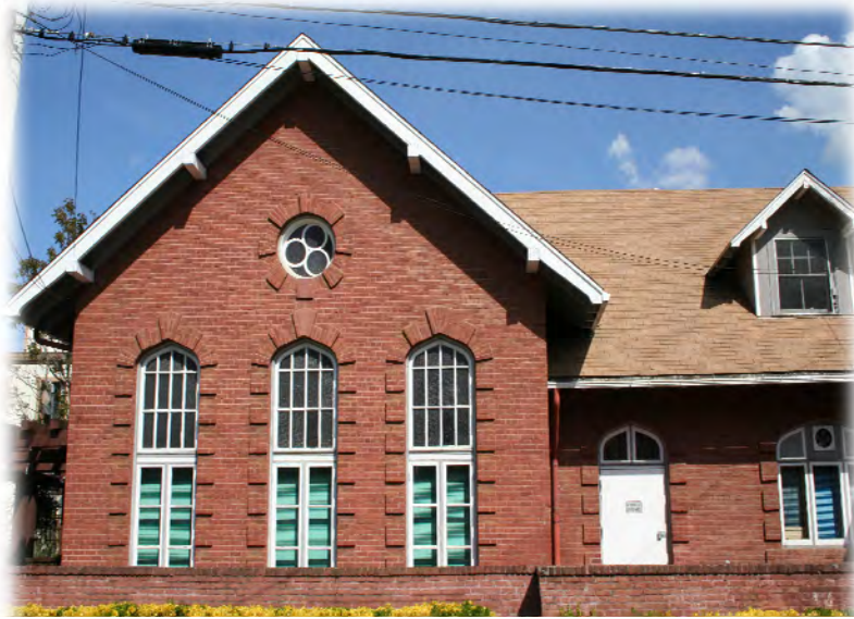
Moderately sloping cross-gable roof applied to a semi-commercial building
