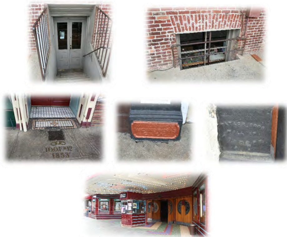
Architectural detail of Grass Valley commercial storefronts: (Top left) Below grade entrance; (Top right) Below grade window detail (Middle left) Ornate tile entry IOOF Hall; (Middle center) Iron pilaster manufactured by Taylor Bros. Machine Works, Grass Valley (Middle right) Cast iron frieze made by Taylor Bros at the base of a pilaster; and (Bottom center) Restored Art Deco Del Oro theater entrance and ticket booth.
