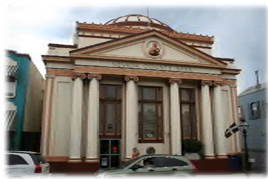
The elegant Neo-Classical Nevada Bank Building.
