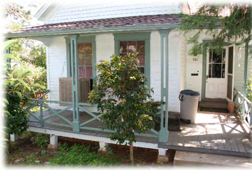
Typical post and pier foundation
