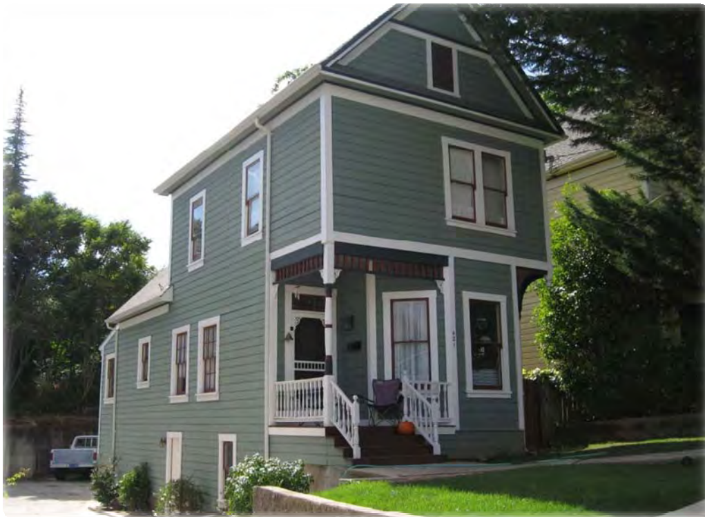
An unusual example of a Late Victorian asymmetric plan, having an inset porch and front gable design bearing Queen Anne architectural elements. A nearly identical house was built upslope on the adjacent parcel.
