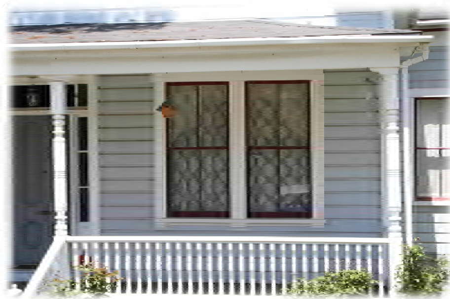
Original paired wood-sash windows with 2 over 2 lights
