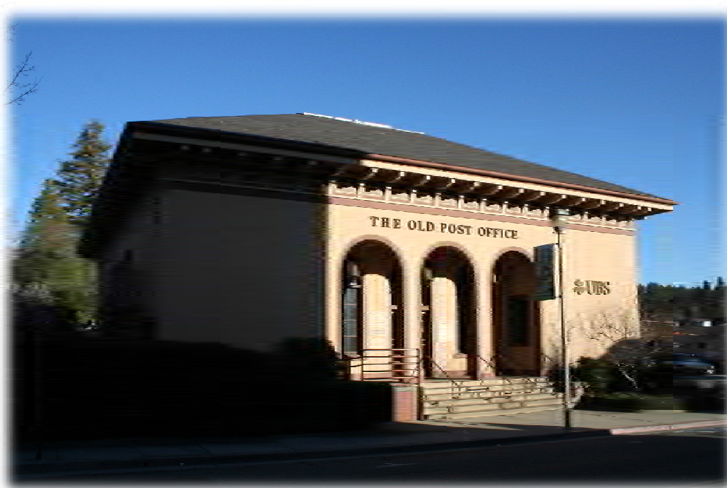
Old Post Office Building on South Auburn Street.
