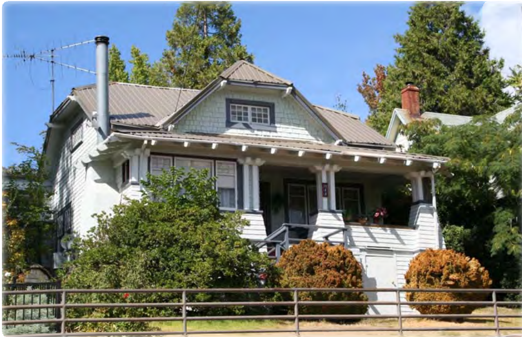
One of the better examples of the true Craftsman or Craftsman Bungalow design. Note the clipped gable roof and multiple porch columns.
