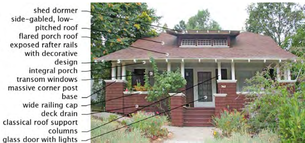
Architectural detail of a Craftsman residence
