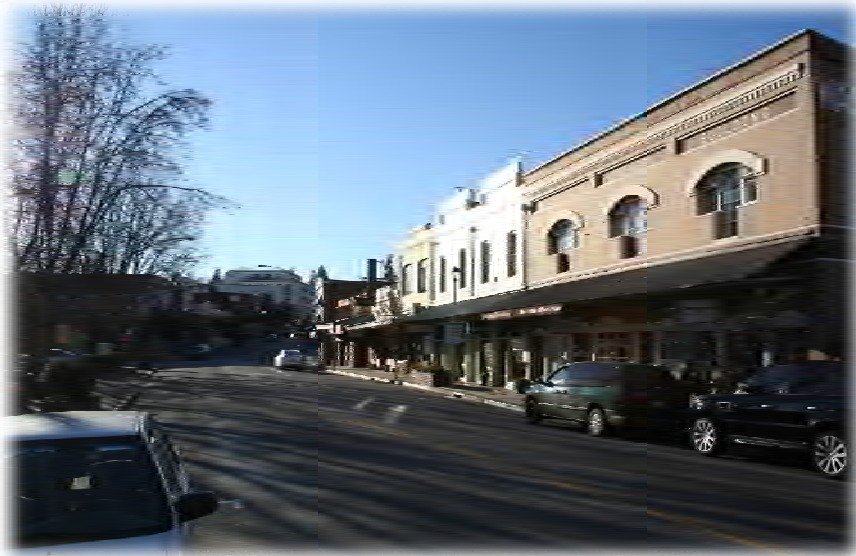
Row of circa 1850s-1860s commercial storefronts with varying recessed entries facing E. Main Street.
