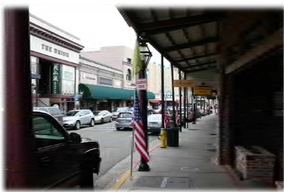
Row of circa 1890s wood and metal roof, and steel column verandas along the west side of Mill Street.
