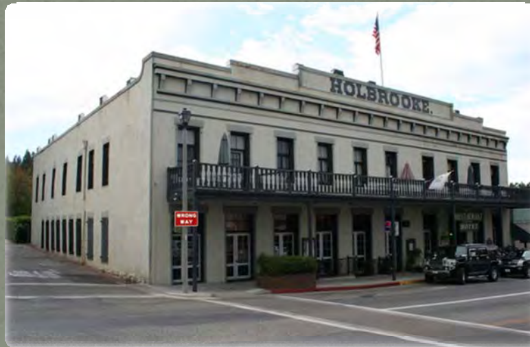
A handsome Classical Revival brick masonry hotel known as the Holbrooke on West Main Street. Note the stepped parapet roof and repetition in the cornice windows and doors.
